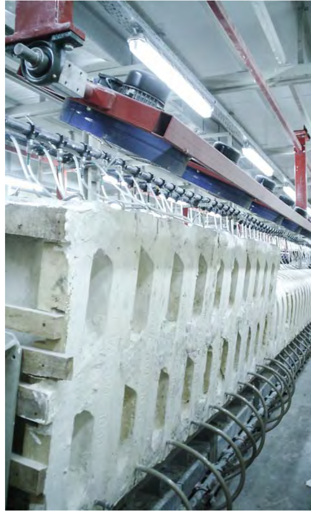
● GNC 1060 Washbasin Casting Plant
