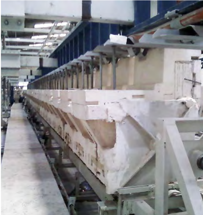
● GNC 1090 Watertank Casting Plant
